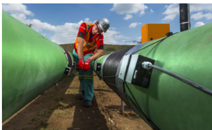
Inspection of fibre optic flow meter installation at Mogalakwena PGMs mine, South Africa.
