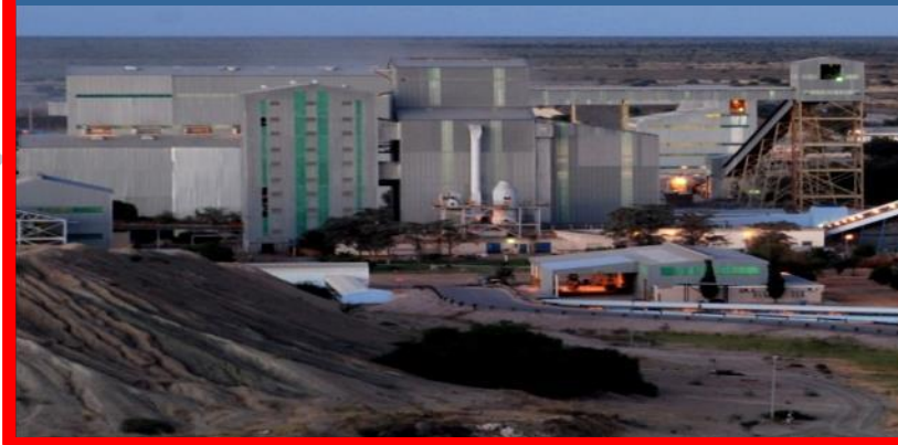
Main treatment plant
