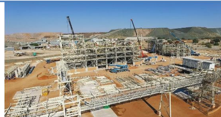
Letlhakane Modular Tailings Plant
