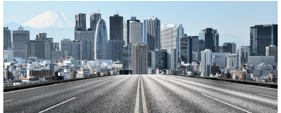
Quality bulks: modern infrastructure development
