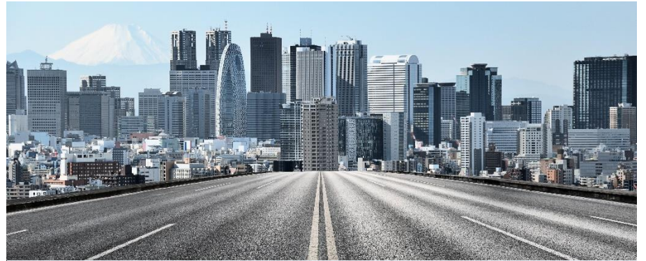
Quality bulks: modern infrastructure development
