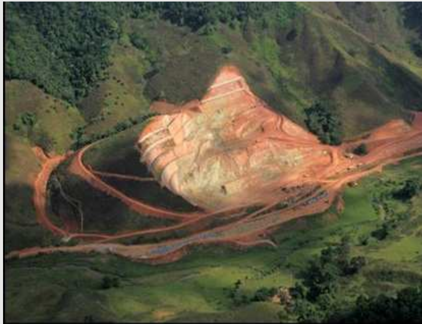
Pump Station #2 Site
