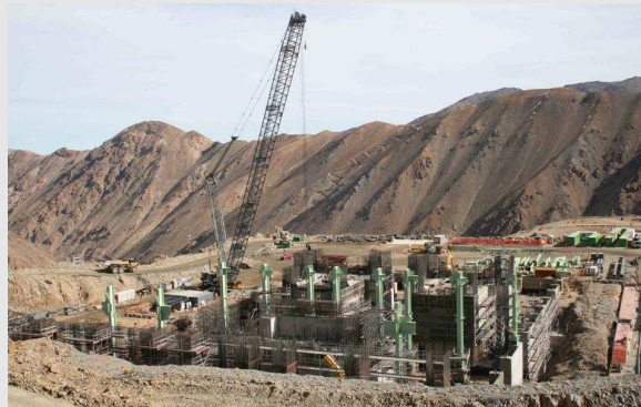
SAG & Ball Mill Foundations at Confluencia
