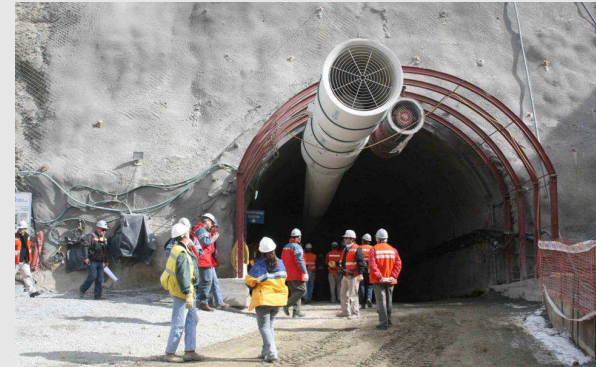
Tunnel to Confluencia
