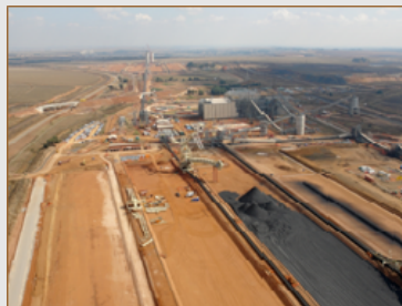
Zondagsfontein mine under construction
