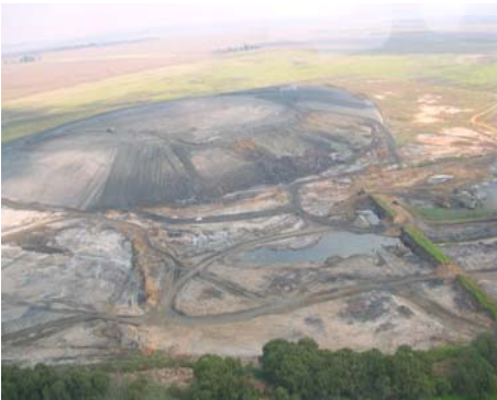
Anglo Coal - Hope Dump during rehabilitation
