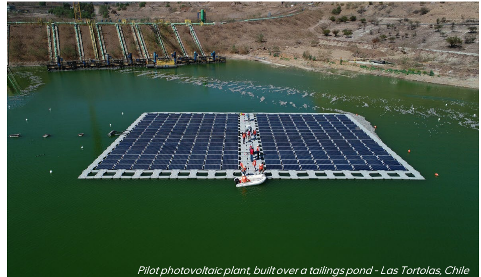
Pilot photovoltaic plant, built over a tailings pond - Las Tortolas, Chile
