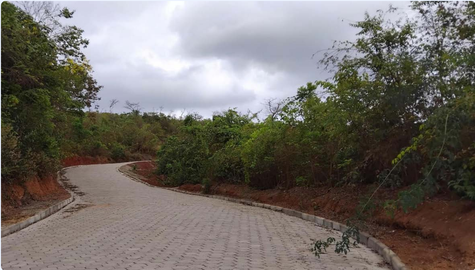
In the neighbourhoods close to Minas-Rio, discarded material from the mine’s processing operations is now being turned into paving blocks for roads, parking lots and pathways.
