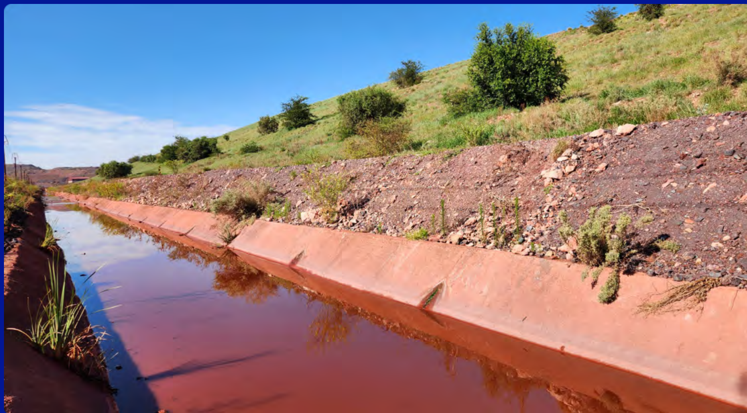
One of the stormwater channels constructed at our Sishen iron ore mine in South Africa to divert excess water away from the mine site.
