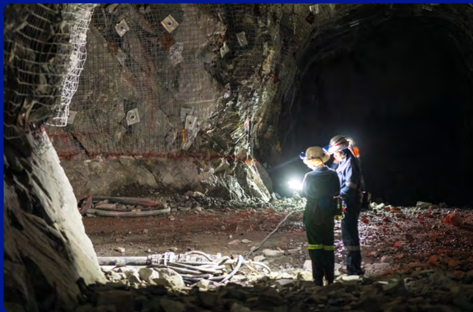
The decline excavation to access underground ore at Mogalakwena, where the installation of high-tensile steel 'blast on mesh' (clearly visible on the stope wall) provides a vital extra layer of protection to development crews.
