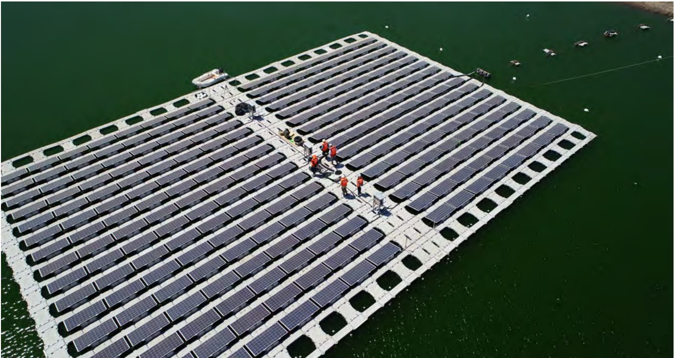
➤ In 2019, at our Los Bronces copper operation in Chile, we launched a pilot photovoltaic plant that has been built over the Las Tórtolas tailings pond – the first of its kind in the world.
