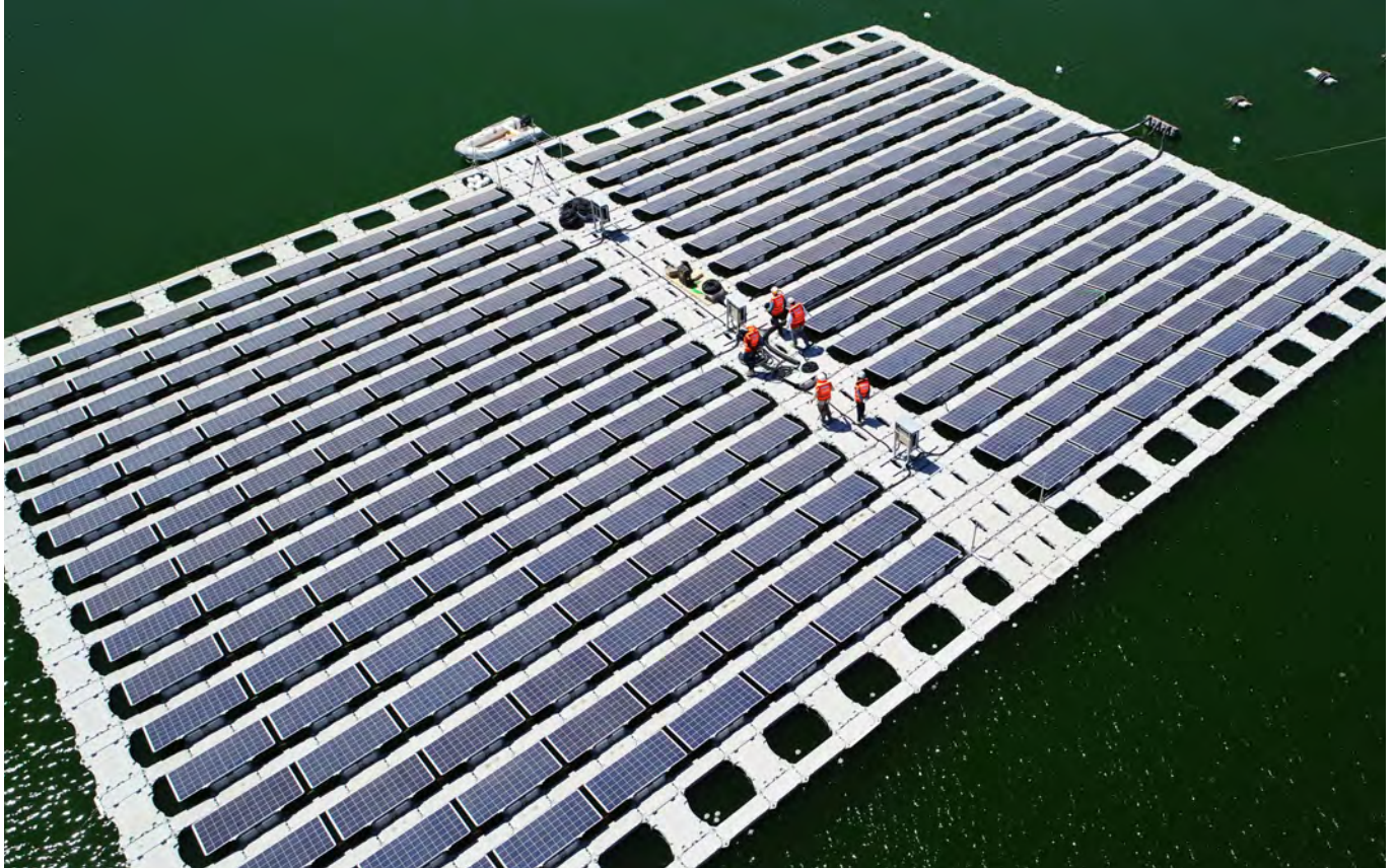
At Los Bronces' Las Tórtolas tailings dam in Chile, a pilot photovoltaic plant built over a tailings pond is the first of its kind. Its 256 panels, located on a floating island, are designed to generate 150,000 kWh of renewable electric power annually and reduce CO 2 emissions by 51 tonnes a year.
