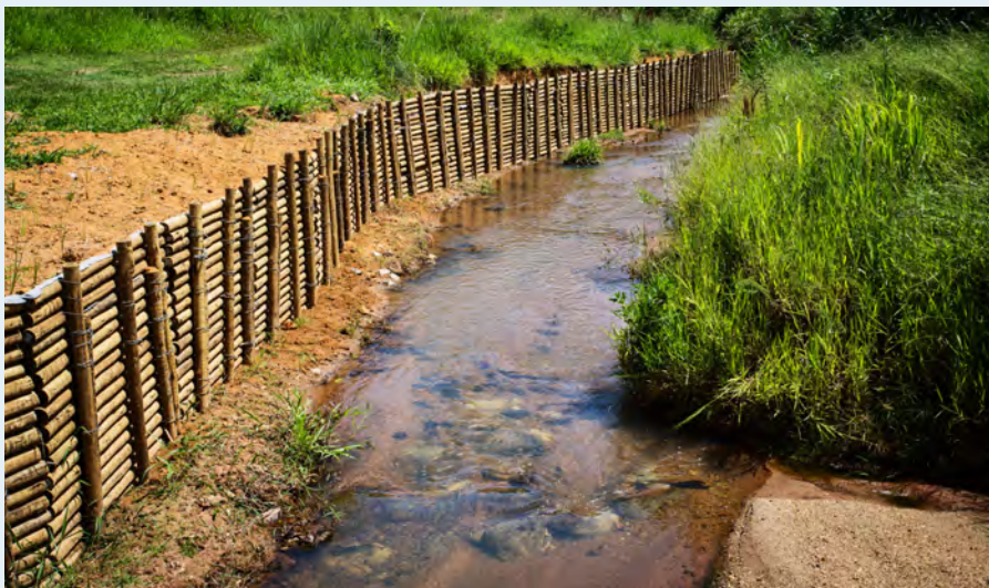
Palisades – a specific type of wooden fence – were built along narrow, curved and other vulnerable stretches of water in order to minimise the effects of water erosion and promote vegetation growth.
