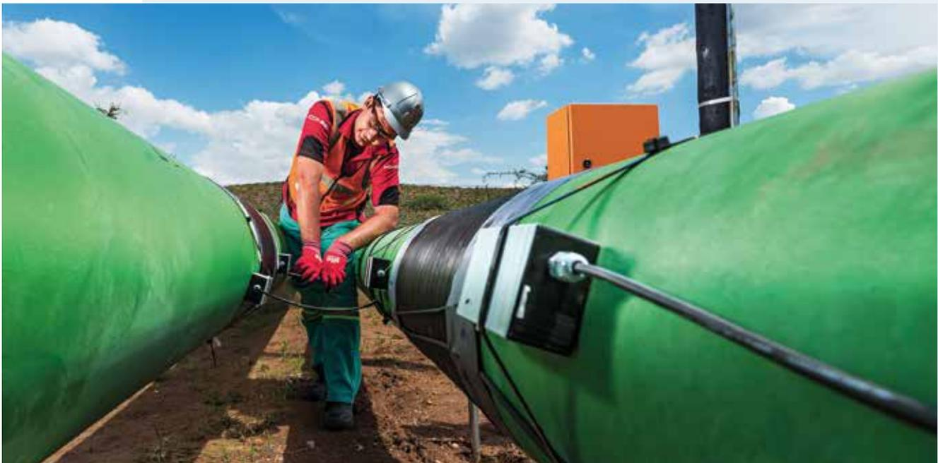
At Mogalakwena platinum mine, in South Africa's water-stressed Limpopo province, technical lead Dean Bothma inspects fibre-optic sensing equipment, enabling accurate, real-time monitoring of all water flows mine-wide. This is the world's first permanent installation using this type of distributed sensing technology.
