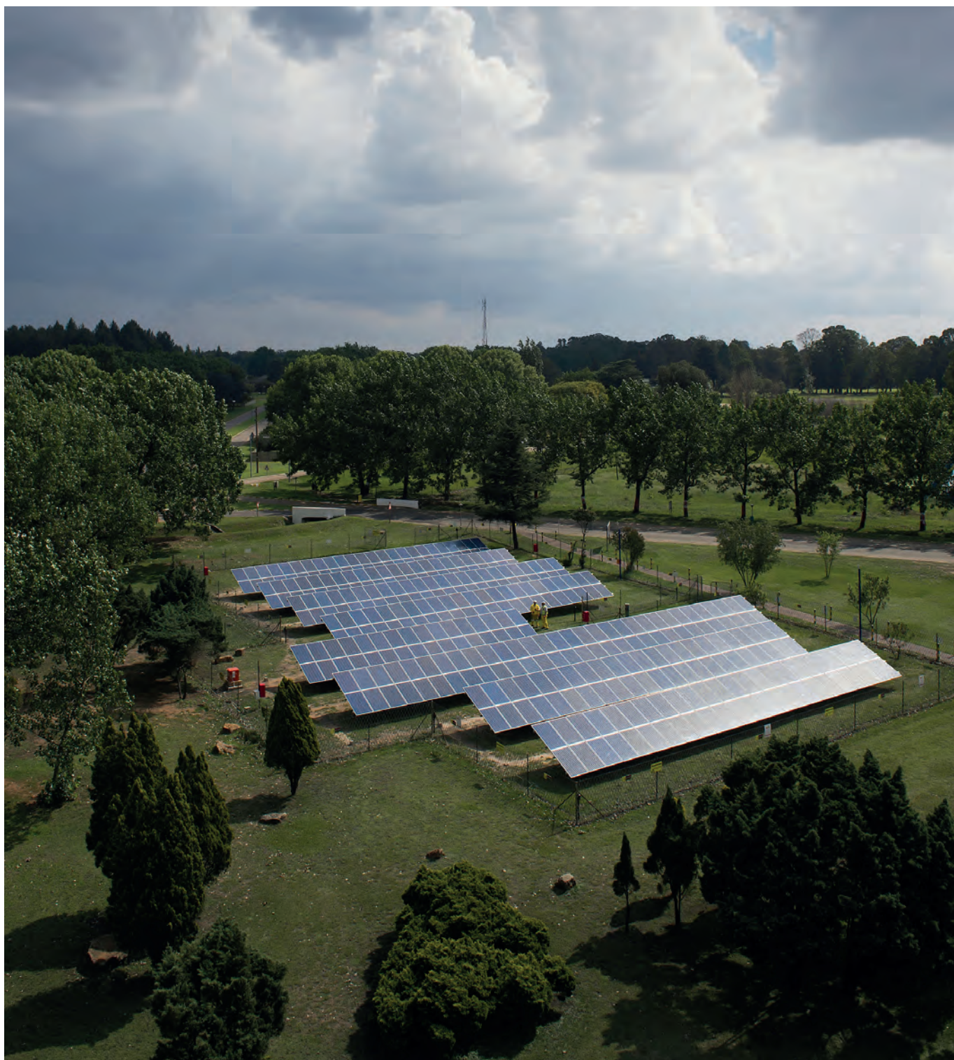
Image: Greenside colliery's solar farm in South Africa consists of 376 photovoltaic panels, adding up to an installed capacity of 90.2 kW at peak.
