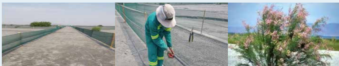
Netting wind barriers being installed and a natural Tamarix shrub on Paardekraal TSF
