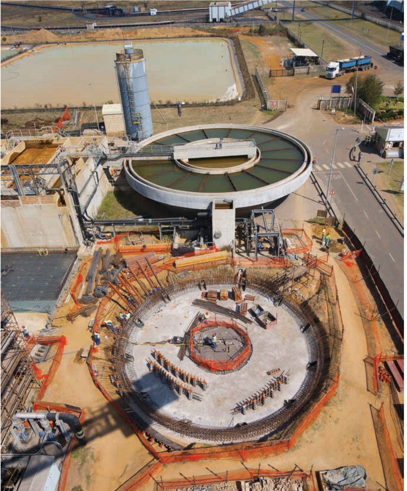
▲ 01 The expansion project at the eMalahleni Water Treatment plant will effectively double the capacity of the plant, drawing waste water from underground workings as far as Landau colliery.
