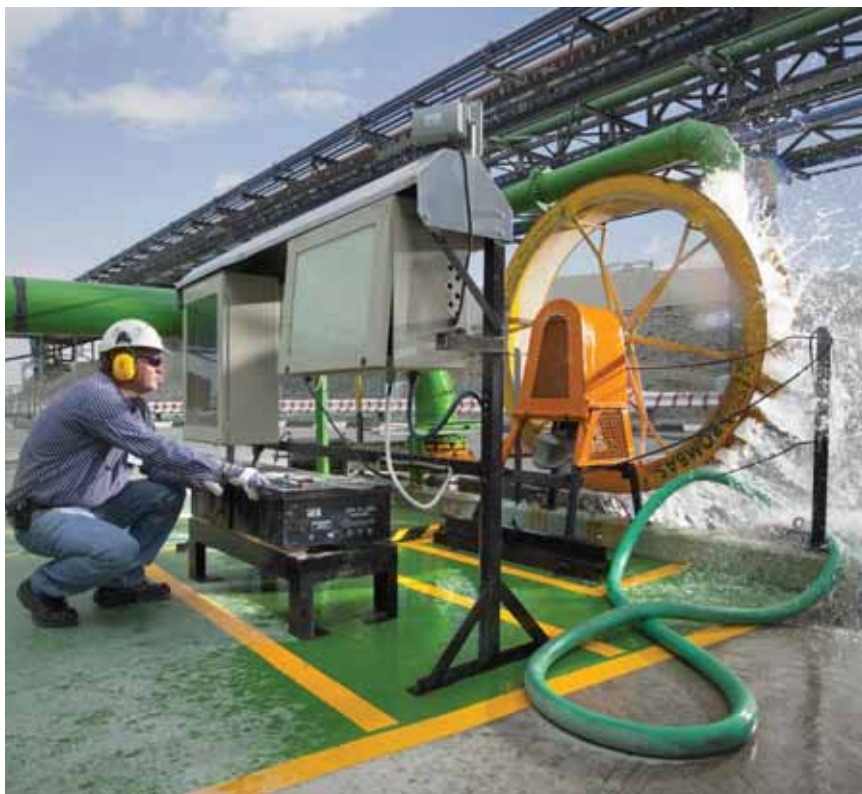
Peet Swanepoel making adjustments to the micro-hydropower generator
