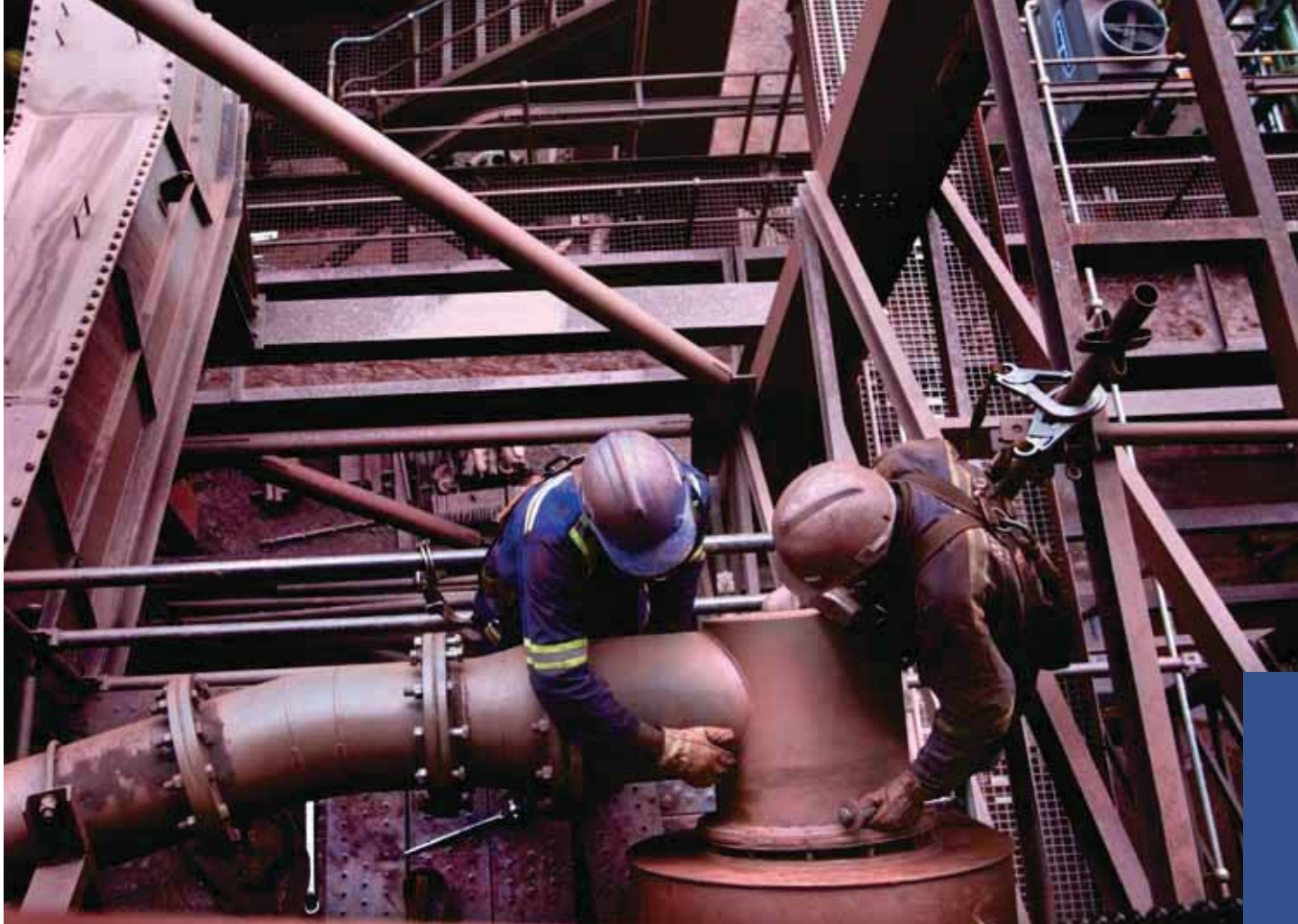
Maintenance workers shifting a pipeline that feeds water to the jig plant at Sishen mine.
