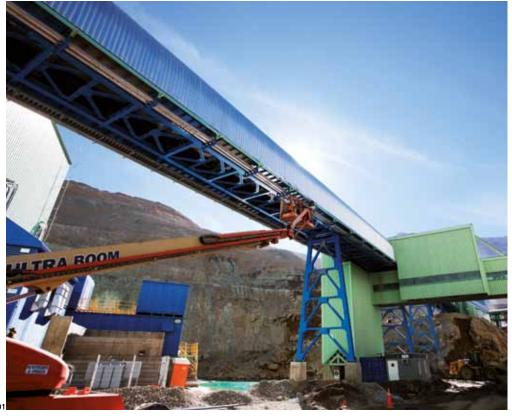
01 In the Confluencia area of Los Bronces, this overland conveyor transports new coarse ore to a stockpile, from where the ore is fed to the SAG mill.
