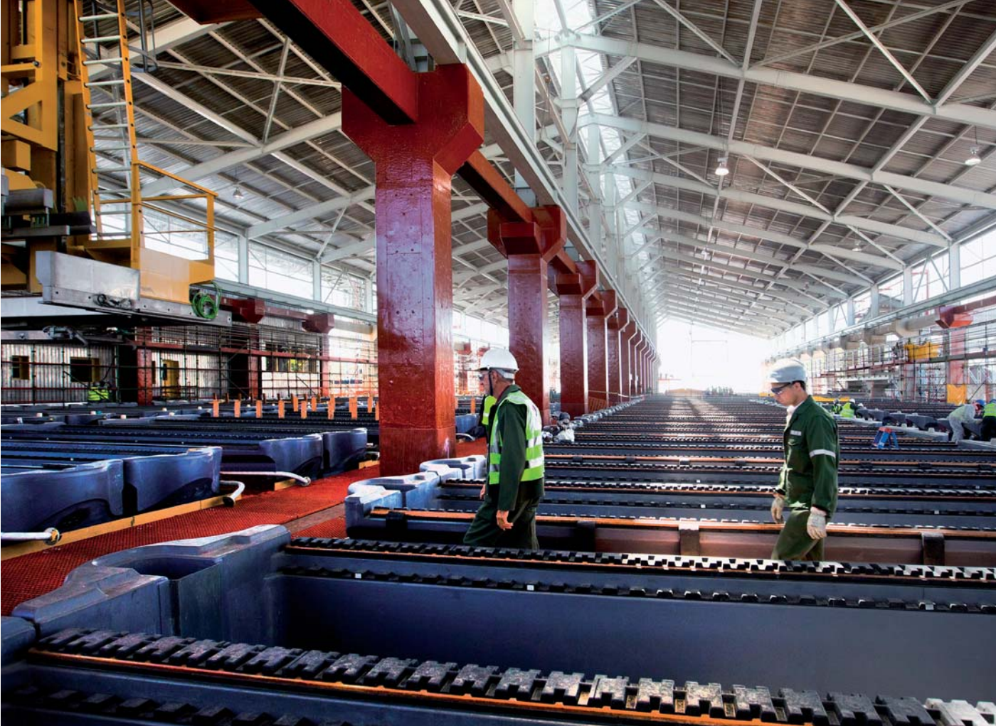
New tank house construction, RBMR.
