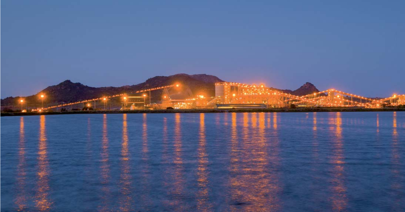
Mogalakwena North Concentrator plant.
