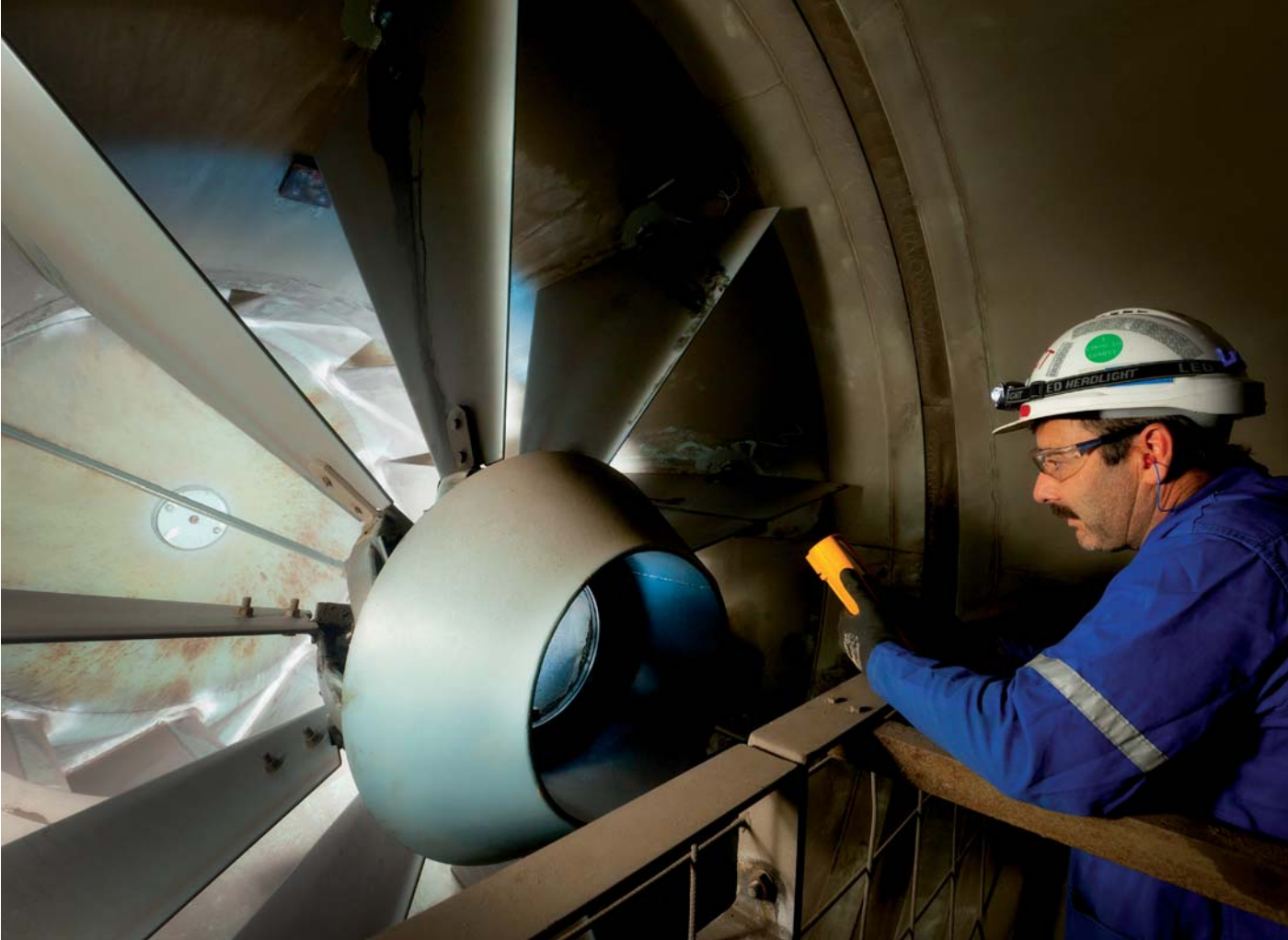
Liam Clelland, an electrician, performs an inspection on the vanes of a ventilation fan.
