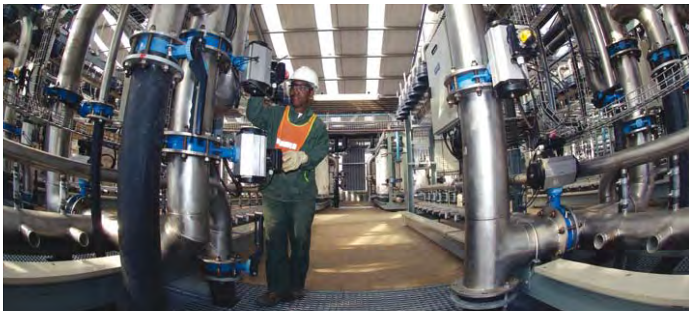
In South Africa, the eMalahleni water-reclamation plant assists in addressing the water demands of the fast-growing eMalahleni area by purifying 25 megalitres of water daily, of which 18 megalitres are supplied to the local municipality
