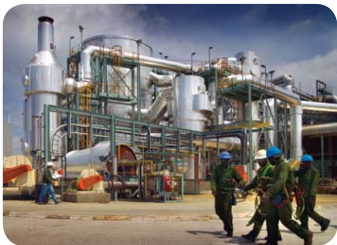
The new double-contact double-absorption acid plant at Waterval Smelter that will allow 99% fixation of sulphur and SO 2 emissions to drop below 20t/day
