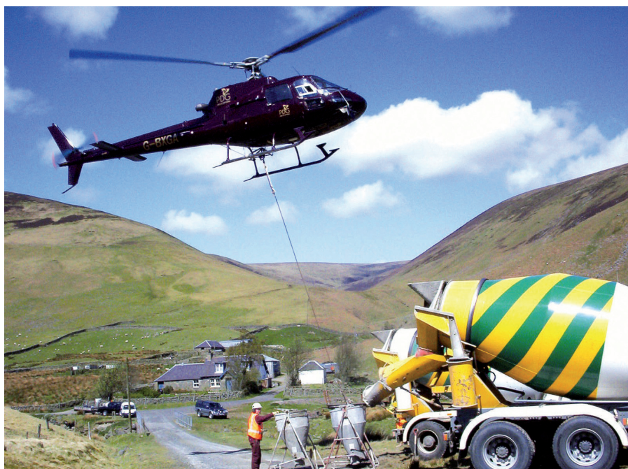
Right: Tarmac concrete takes the high road in Scotland as concrete is airlifted to instal a phone mast
