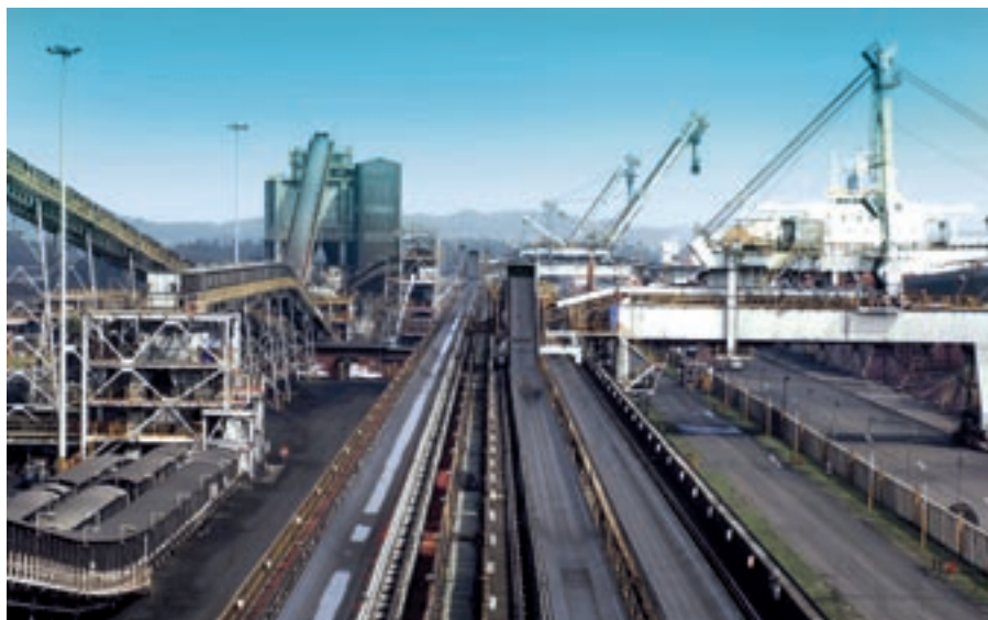
Right: View of the quay and massive conveyor system which transports coal to the ships at Richards Bay Coal terminal in South Africa
