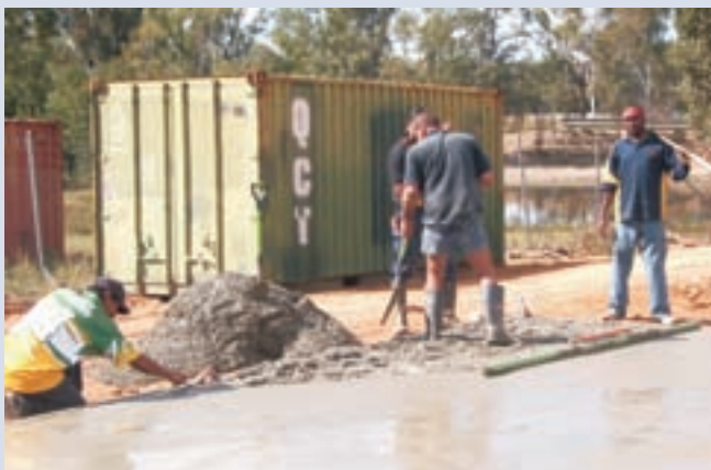
Dale Burden from Capcoal mine helping workers to lay the concrete slab for the timber products work area.
