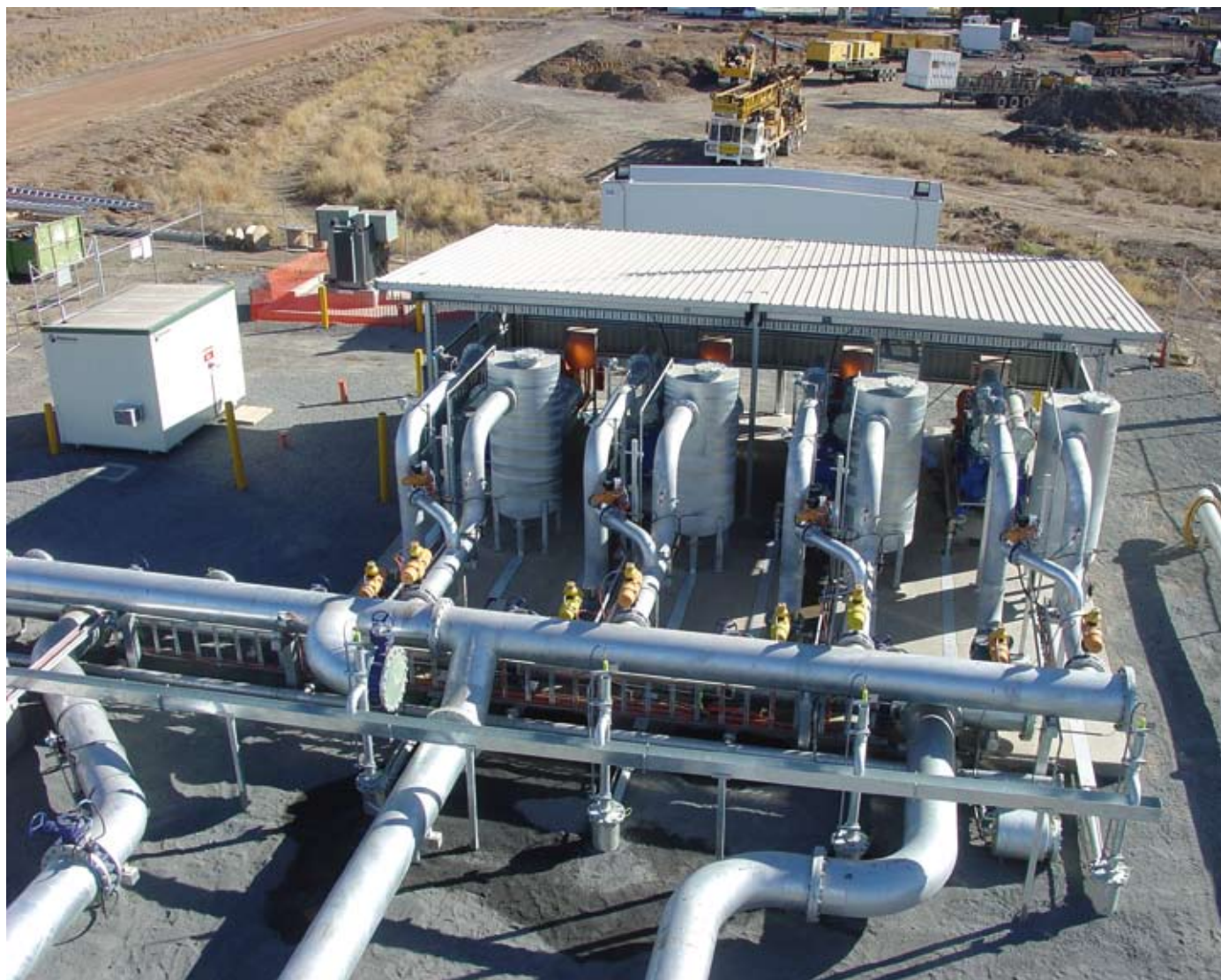
The Capcoal 32-megawatt coal seam methane-fired power plant which reduces Anglo Coal's greenhouse gas emissions by 1.1 million tonnes of CO 2 e per year
