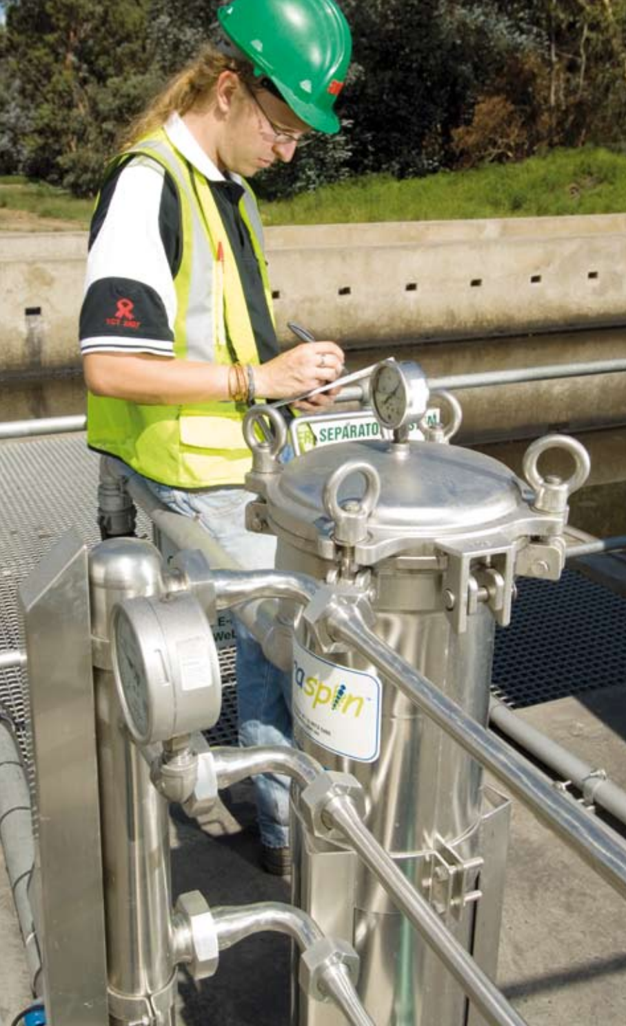
Environmental officer Milton Milaras inspects New Vaal colliery's newly-installed oil and silt separator, which has dramatically improved the mine's clean and dirty water separation
