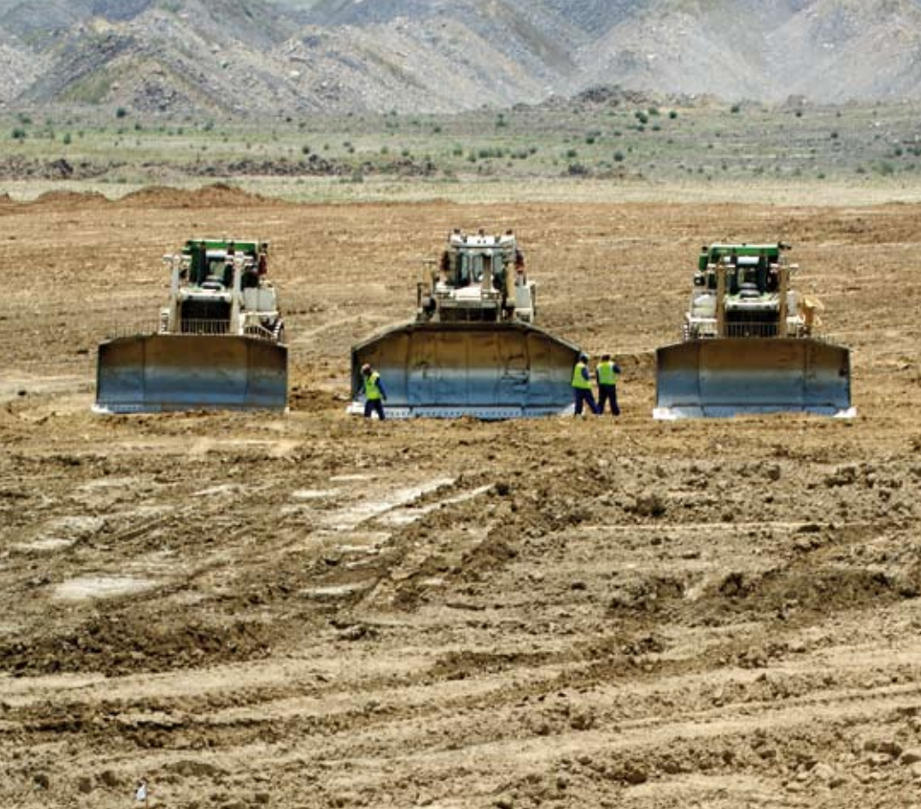
Land rehabilitation in progress – the process includes levelling of open-cast mine spoil heaps to original surface contours.
