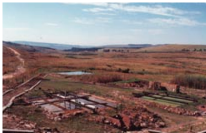
Passive water treatment pilot plant at Vryheid Coronation colliery in KwaZulu-Natal
