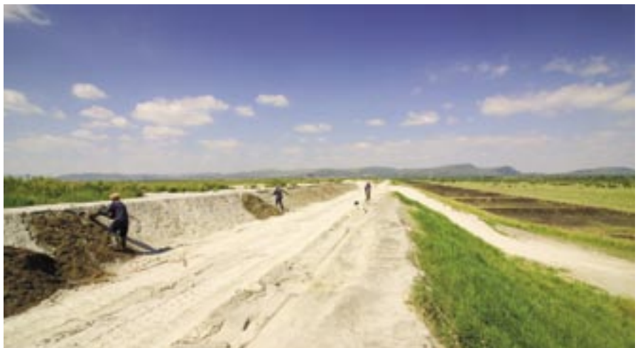
Compost from sewage sludge and woodchips applied to the BRPM tailings dump.
