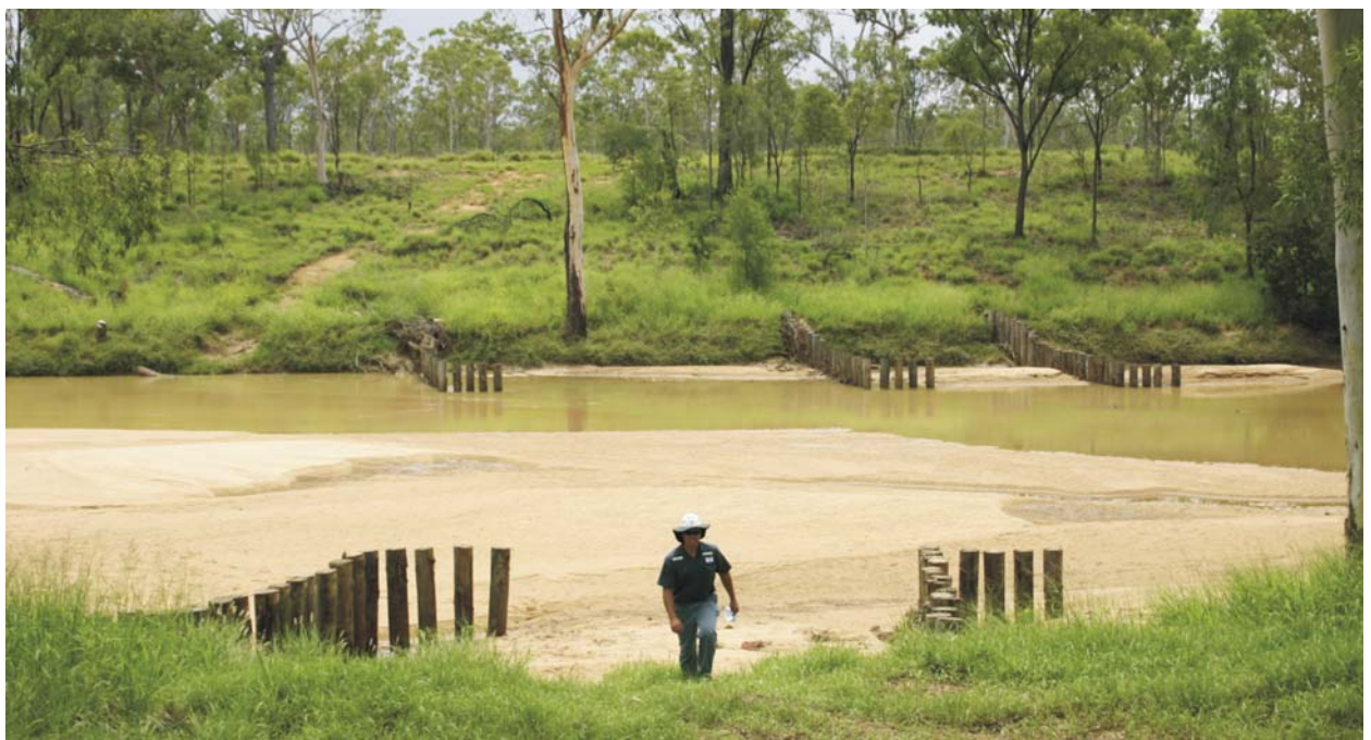
Environmental Graduate, Tom Hayes, inspecting a section of the Isaac River subsidence stabilisation works after rain and associated river flows.
