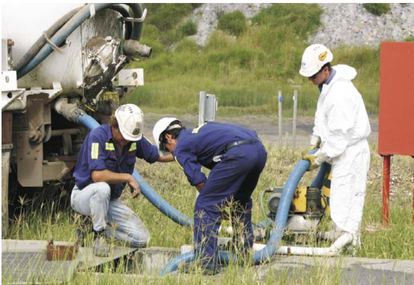
Contractors (from left) George Thrift and Daniel Wisemantel assist Paul Tierney in removing waste sludge from workshop drains and washpad sumps.
