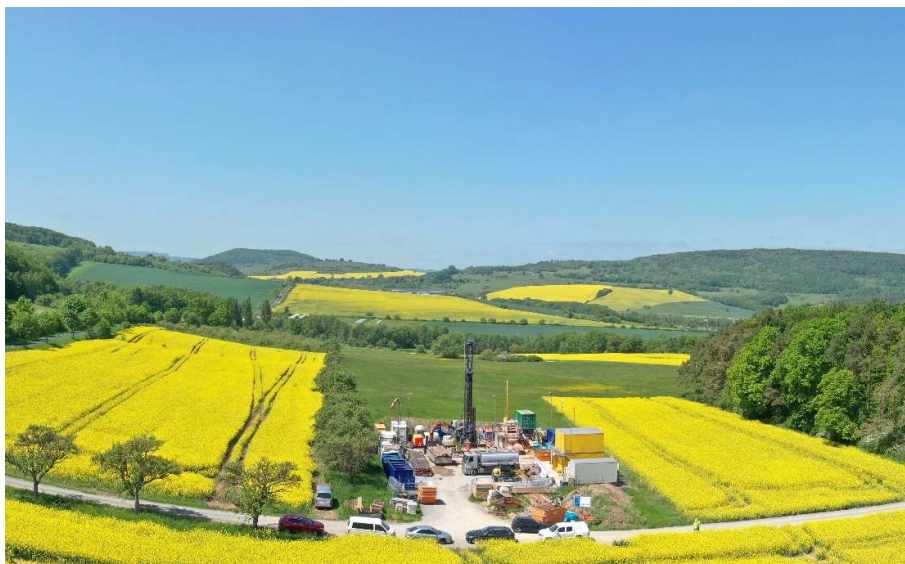
Drillsite with drilling rig for exploring the copper shale near Unterkatz, southern Thuringia
