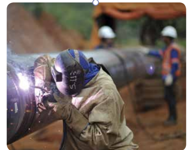
Welding a section of the 529-kilometre pipeline that transports iron ore in slurry form to the Port of Açú
