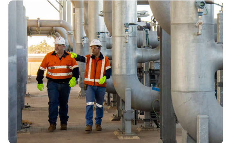
Gas plant at Grosvenor. Around 60% of the methane gas from our underground coal mines is captured and then supplied to Queensland's electricity grid.
